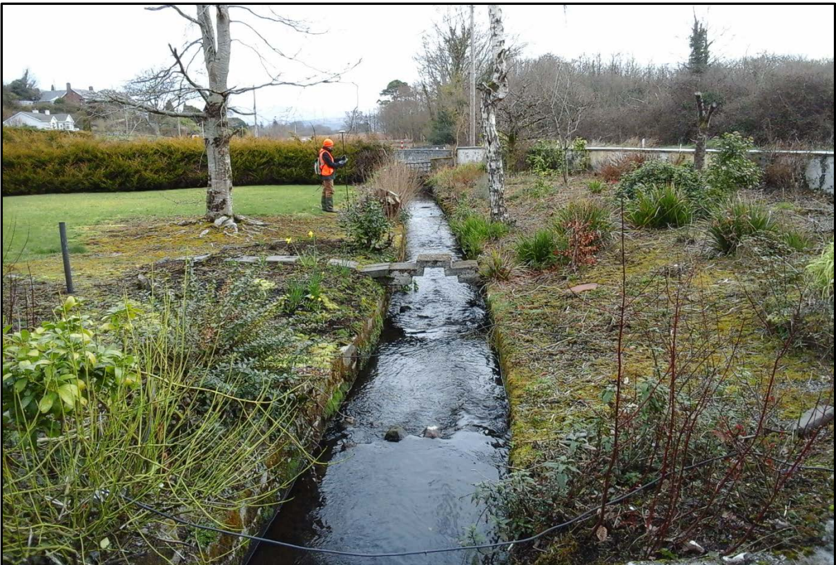
Photograph 24: Reach 5 (looking downstream from bridge at Judge's residence)
