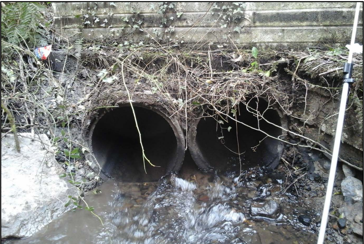
Photograph 12: Culvert 3 (downstream end)
