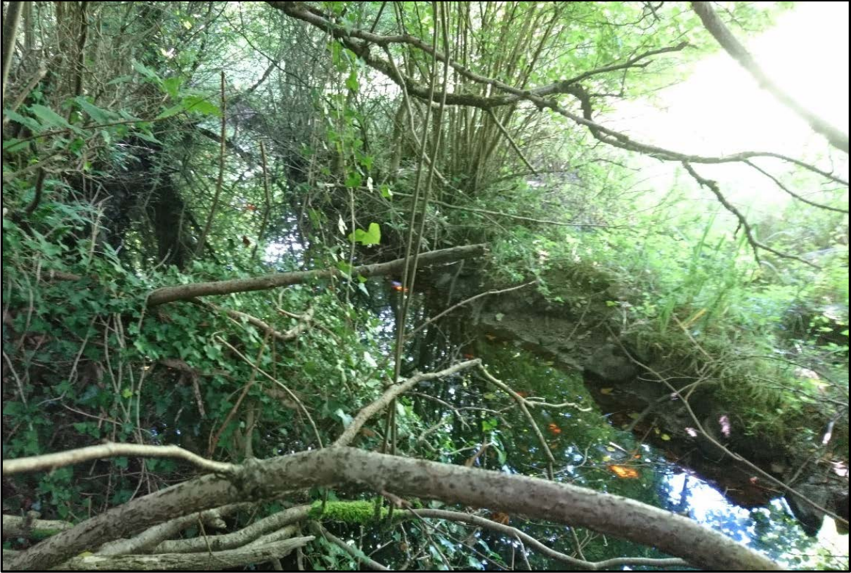
Photograph 1: Upstream of Culvert 1 (looking upstream)
