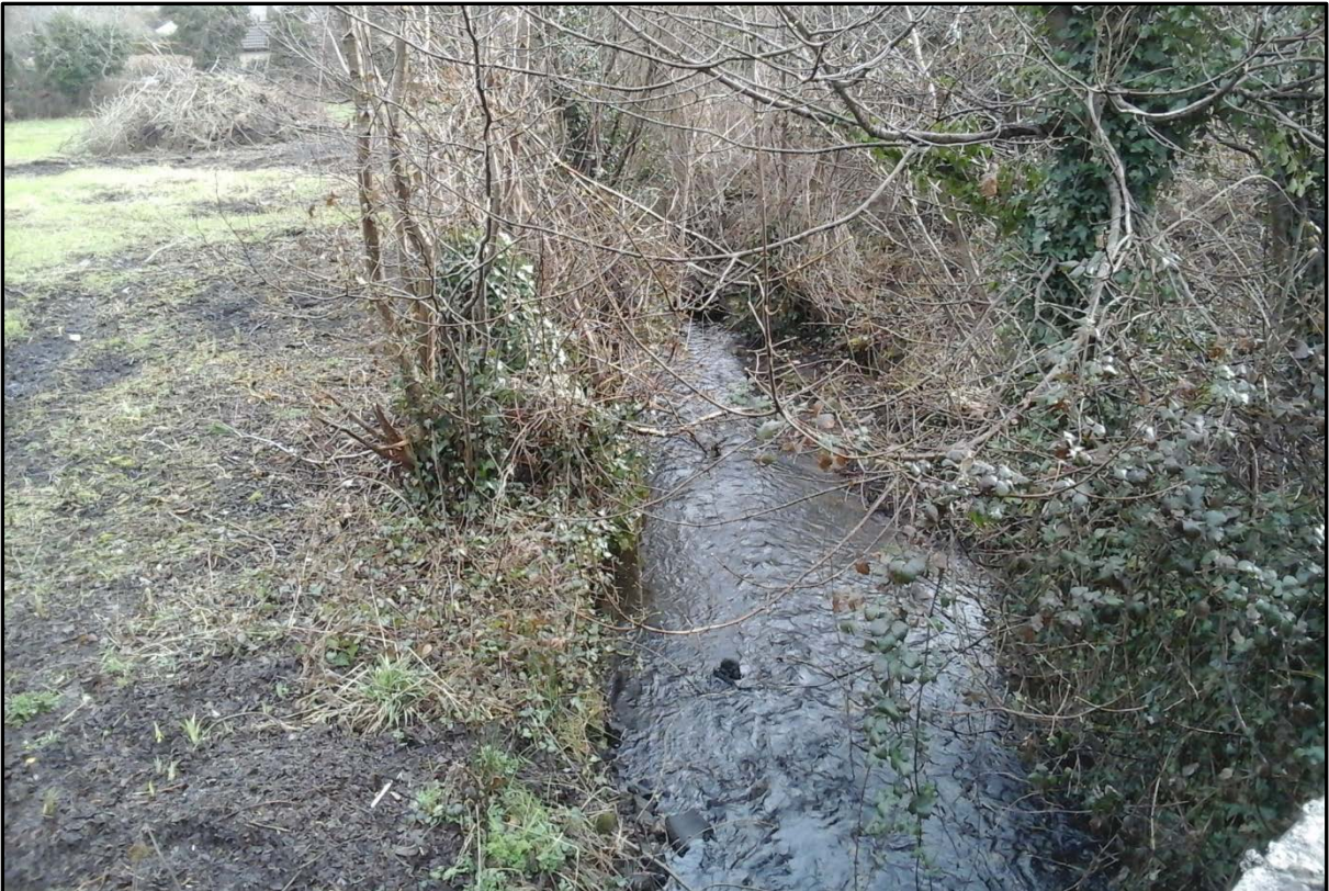
Photograph 22: Reach 5 (looking downstream from bridge at Culvert 5)
