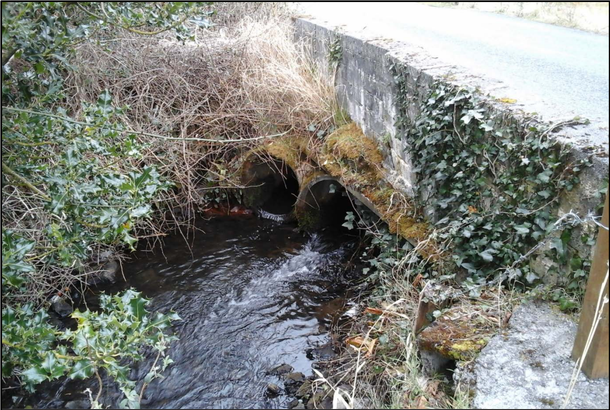
Photograph 27: Culvert 6 (downstream end)
