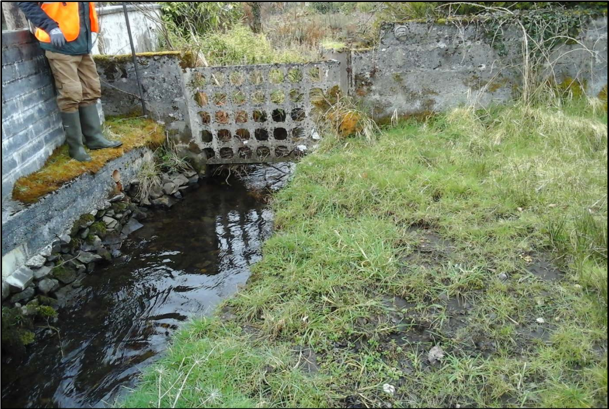
Photograph 25: Reach 5 (looking upstream at Culvert 6) – Note perforated concrete fence over stream
