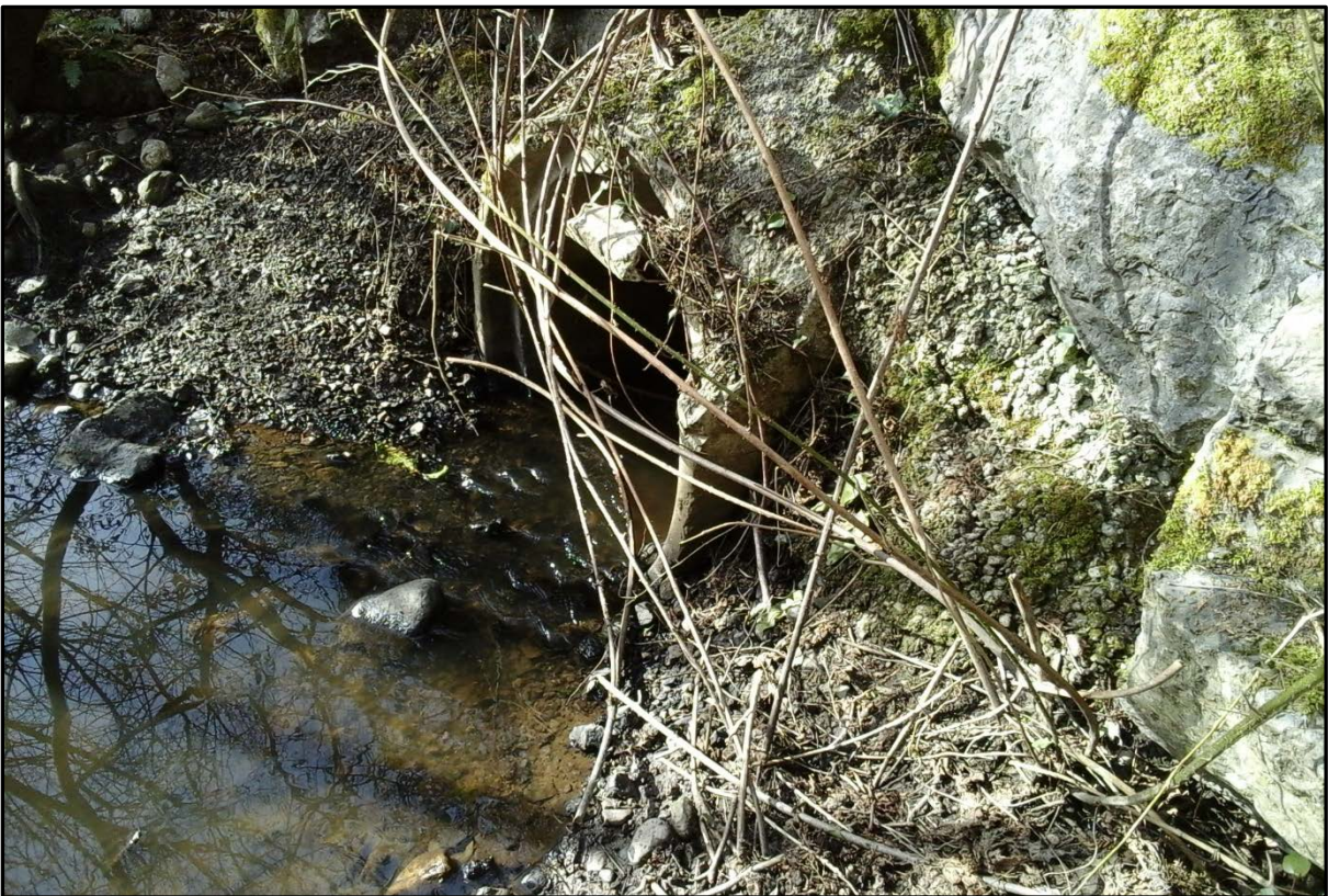
Photograph 2: Culvert 1 (upstream end)
