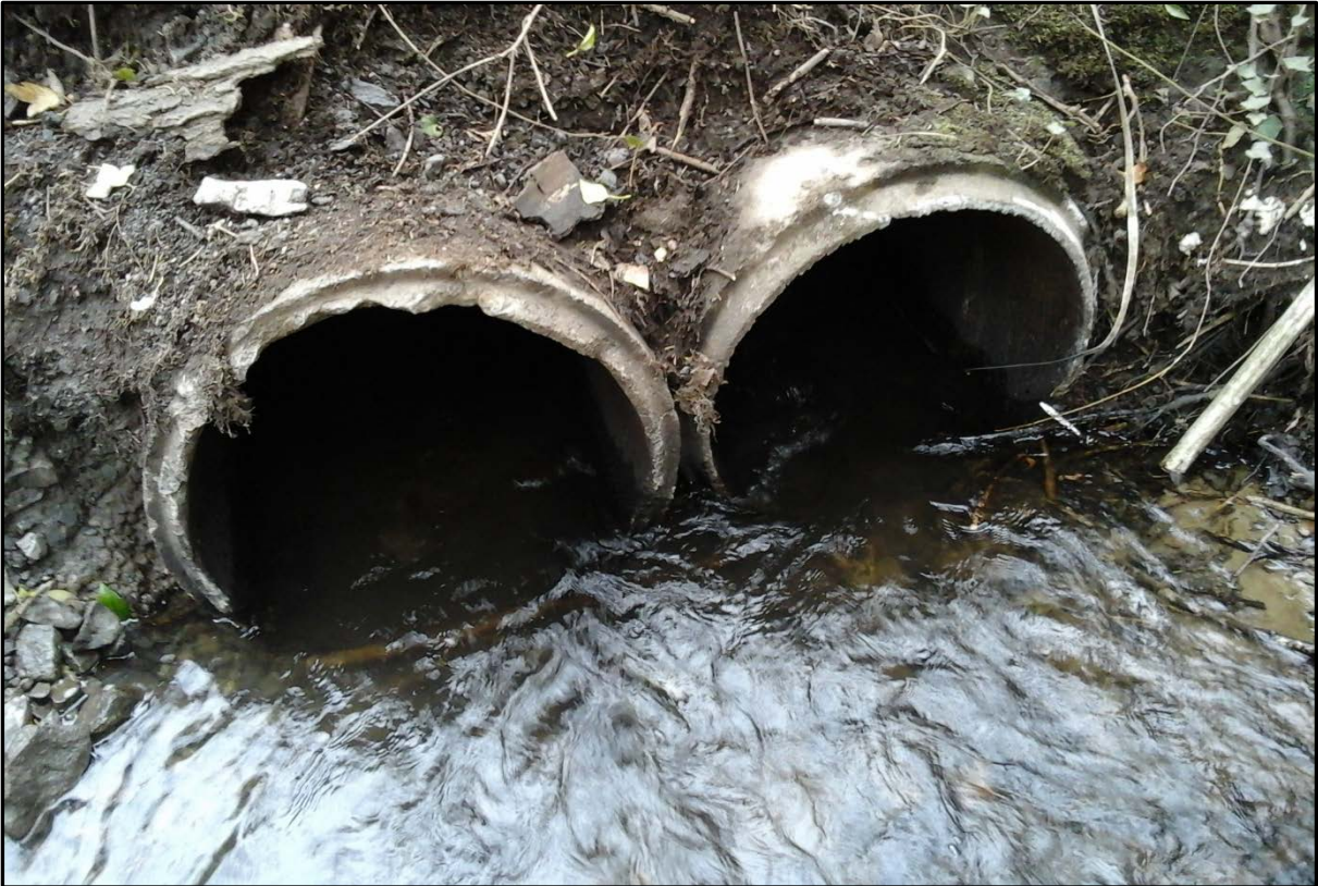
Photograph 11: Culvert 3 (upstream end)
