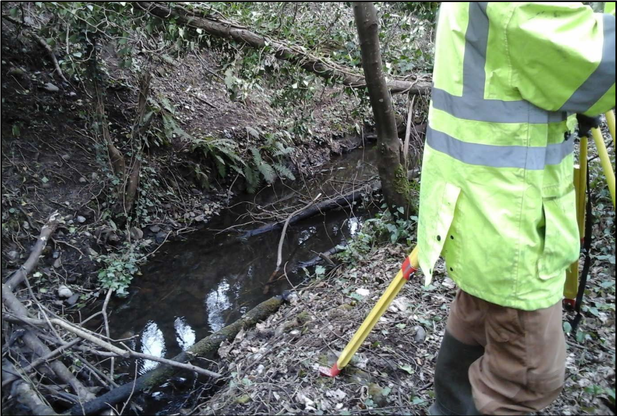
Photograph 7: Reach 1 (looking downstream, approaching Culvert 2)
