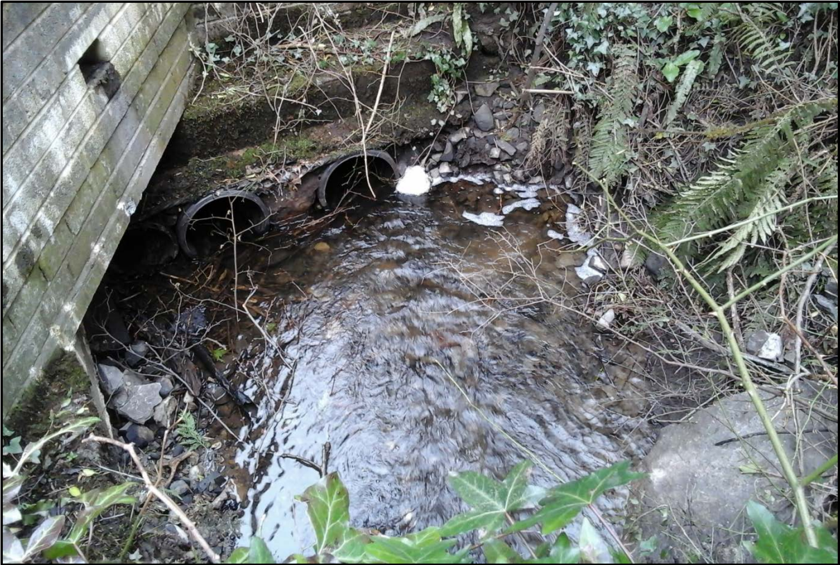
Photograph 13: Reach 3 (looking downstream) – Note concrete brick wall surrounding reach
