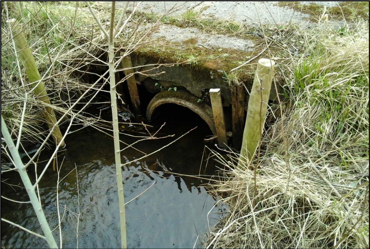
Photograph 29: Culvert 7 (upstream end)
