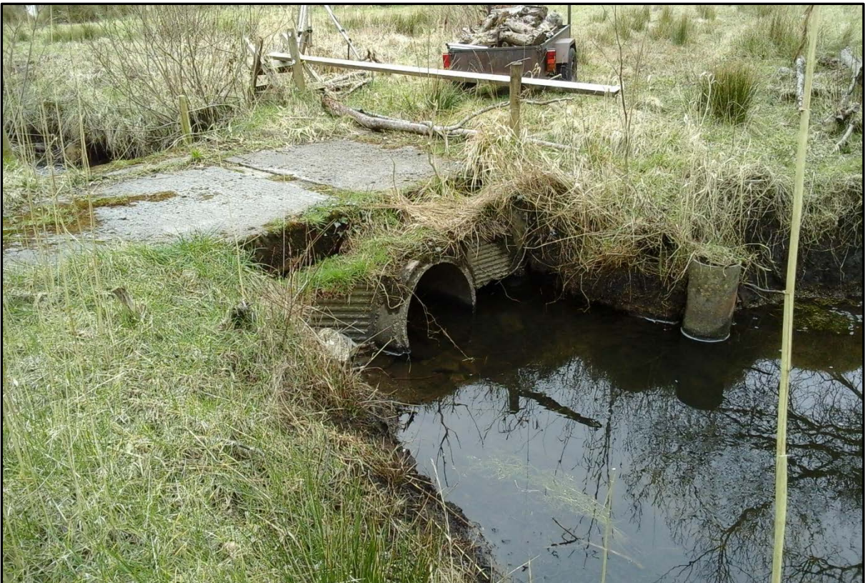
Photograph 30: Culvert 7 (downstream end)
