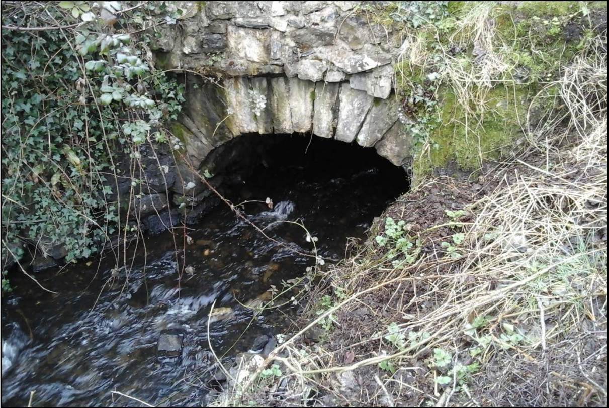
Photograph 21: Culvert 5 (downstream end)
