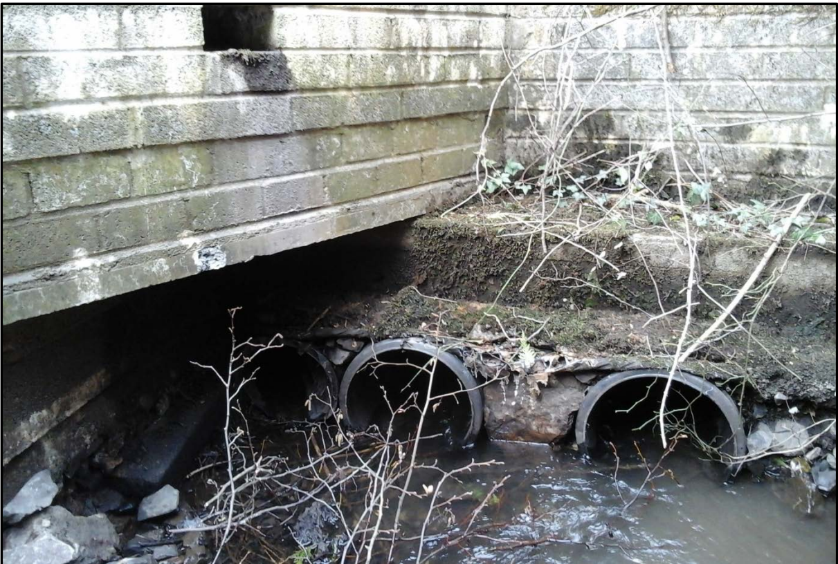
Photograph 14: Culvert 4 (upstream end) – Note smaller pipe on left diverts water to private pumphouse
