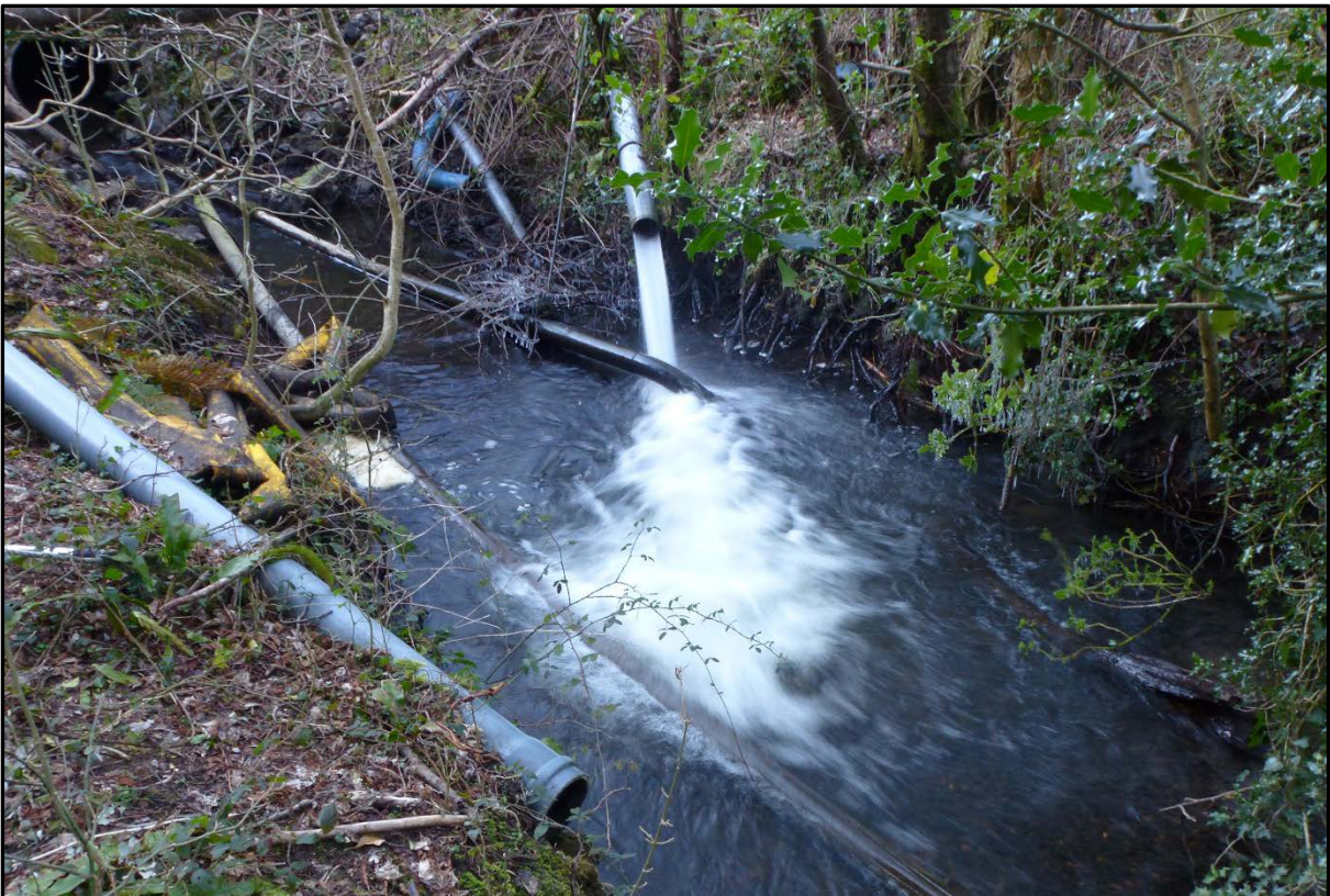
Photograph 4: Reach 1 (looking upstream) – Note two quarry discharge pipes, one discharging
