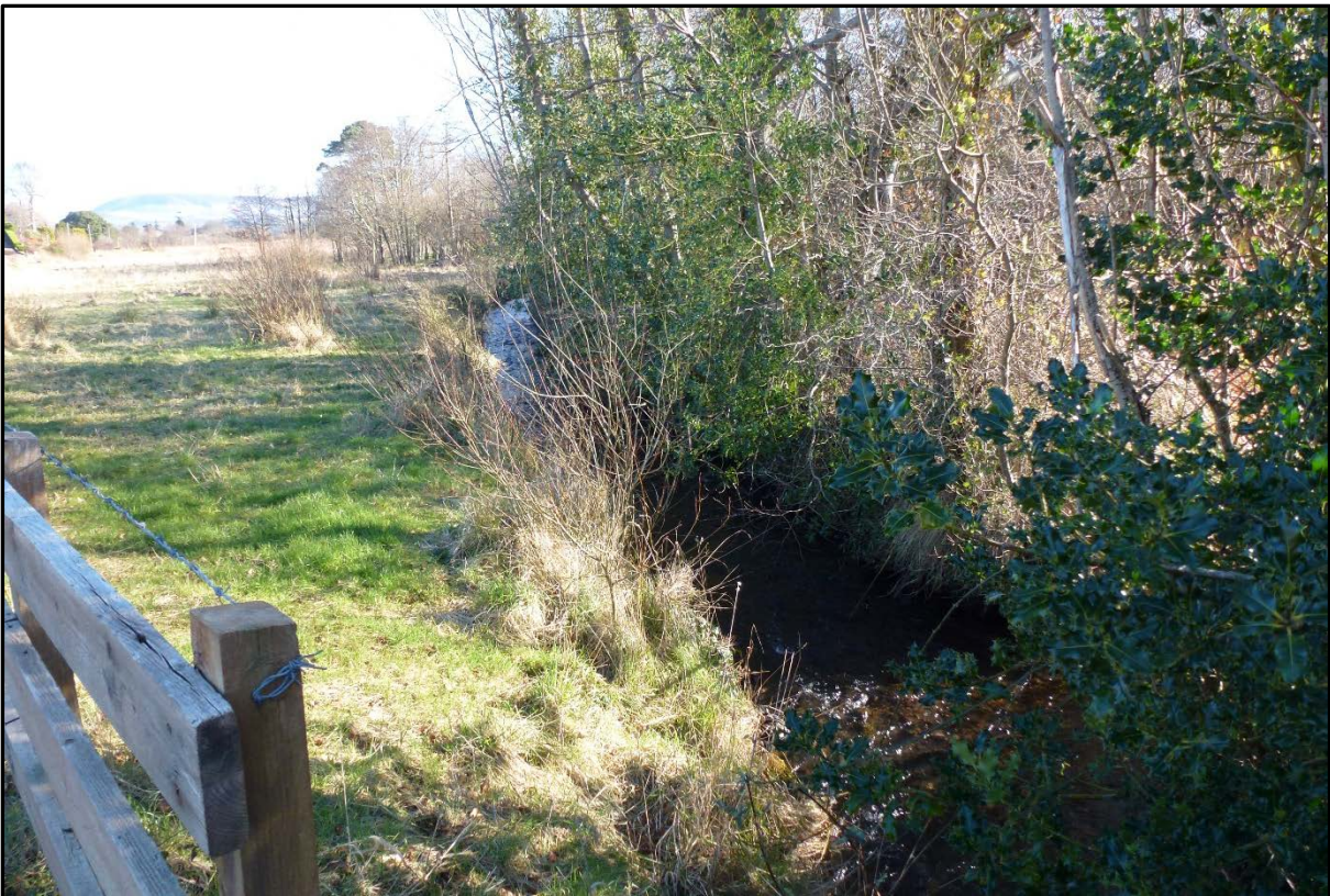
Photograph 28: Reach 6 (looking downstream from bridge at Culvert 6)
