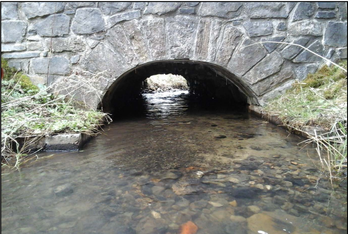
Photograph 20: Culvert 5 (upstream end) – Arched culvert under main public road R287
