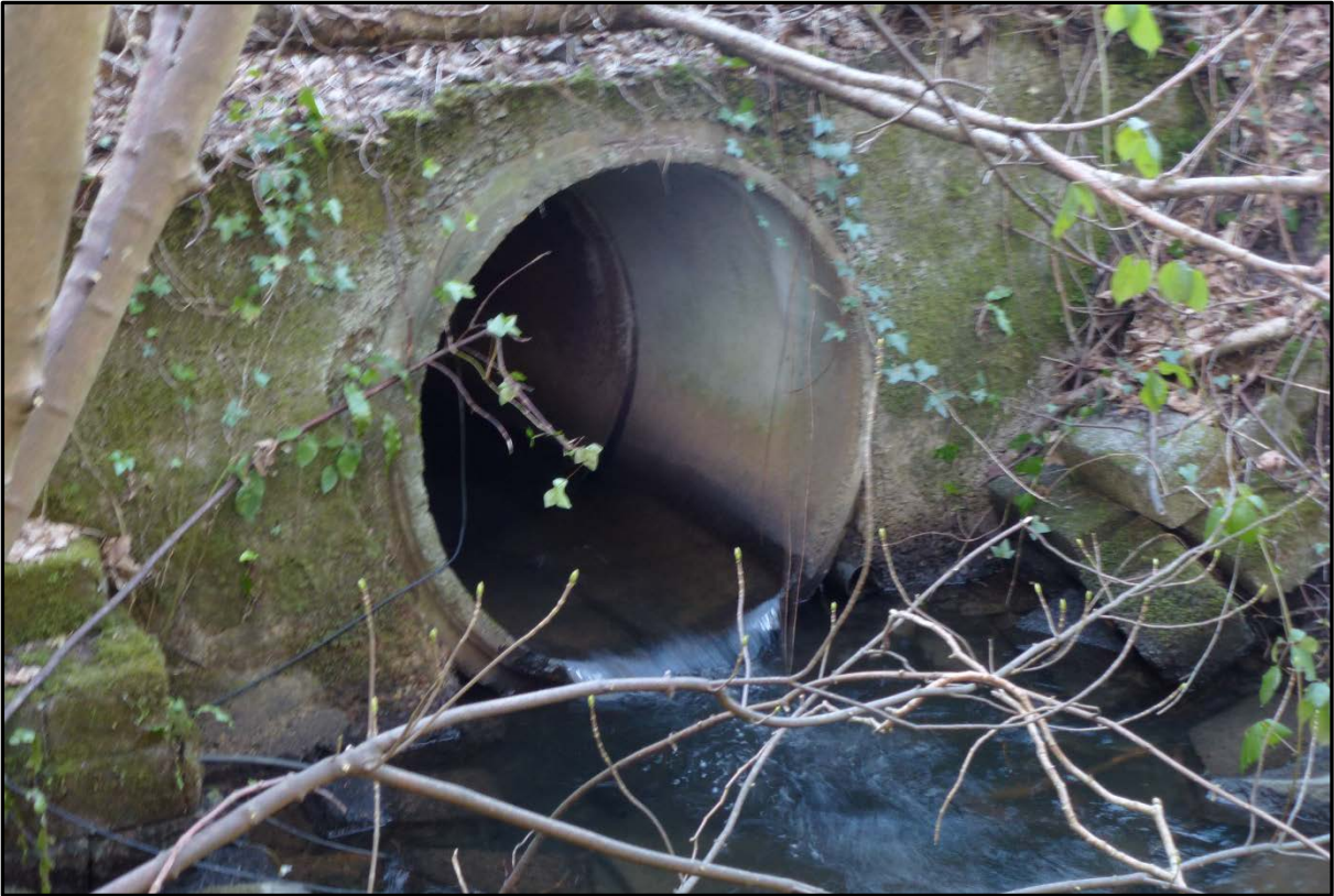
Photograph 9: Culvert 2 (downstream end)
