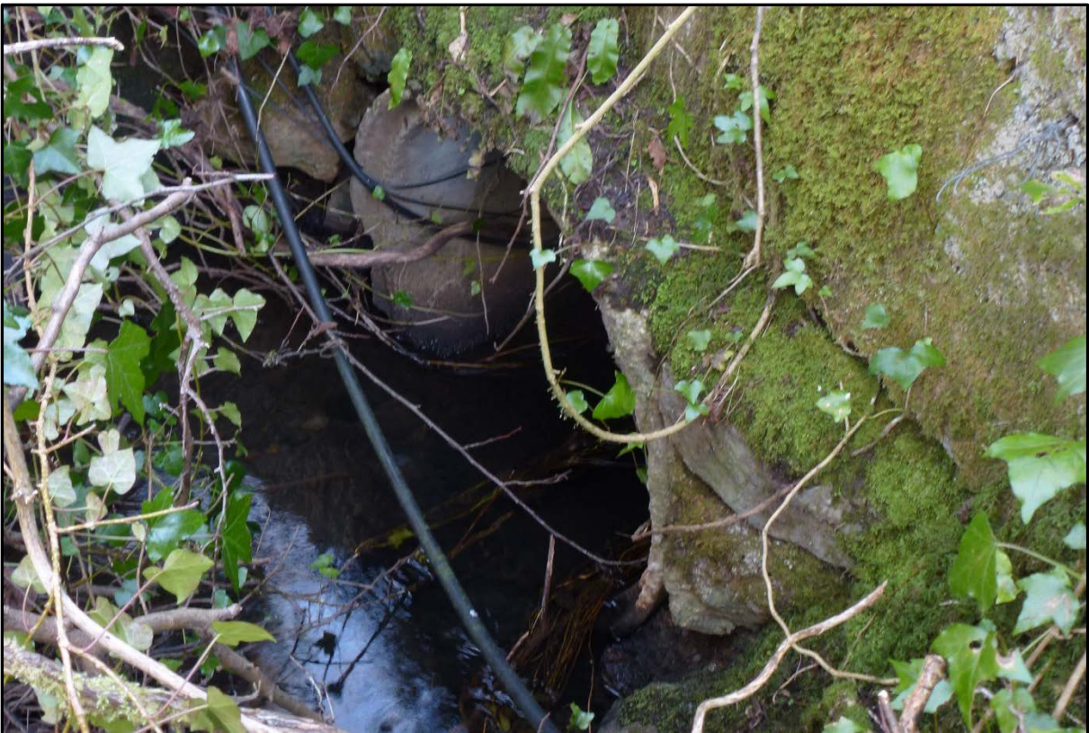
Photograph 8: Culvert 2 (upstream end)
