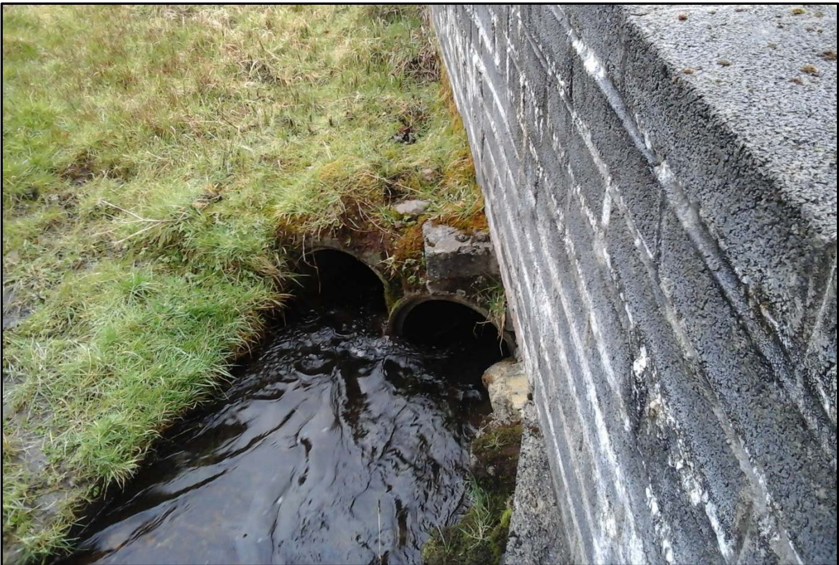
Photograph 26: Culvert 6 (upstream end)
