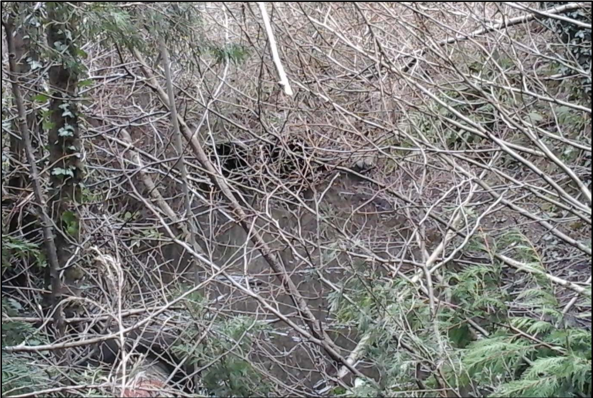
Photograph 15: Culvert 4 (downstream end) – very overgrown on banks
