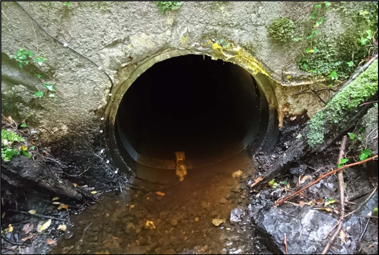
Photograph 3: Culvert 1 (downstream end) – Note Starflow flowmeter installed
